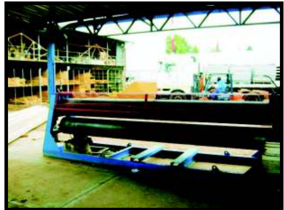
Truss Factory Equipment
