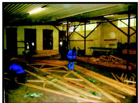
Truss Assembly Plant
